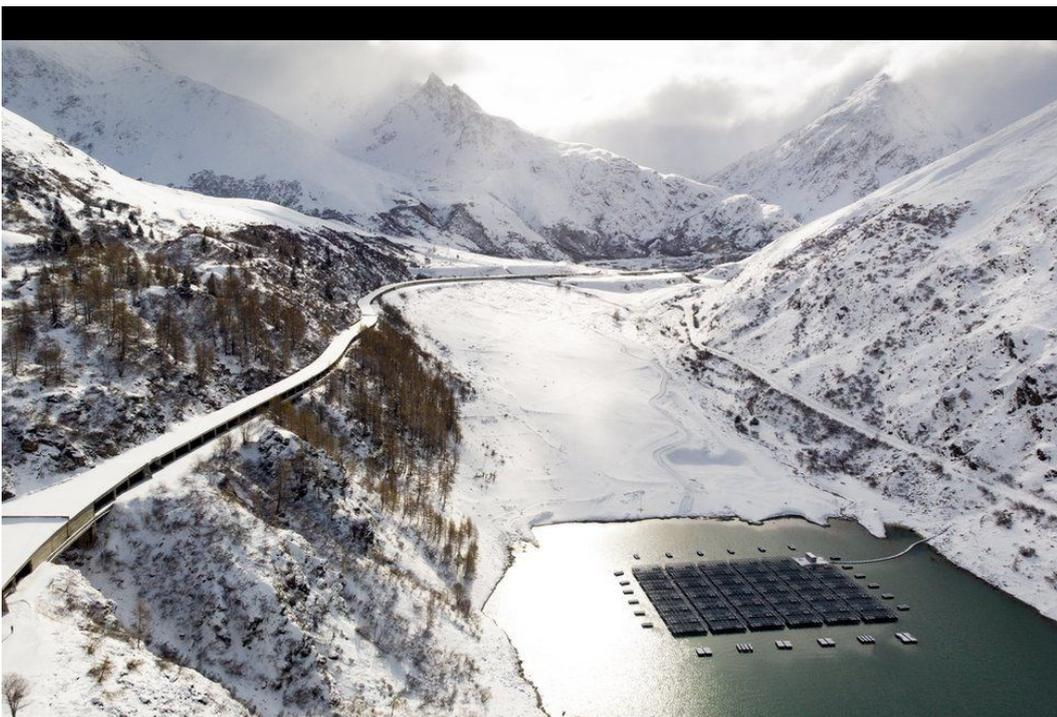
*Floating barges with solar panels on the Lac des Toules, an alpine reservoir lake in Bourg-Saint-Pierre, Switzerland. The floating solar panel station consists of 36 floating barges featuring 2,240m<sup>2</sup> of solar cells.*
